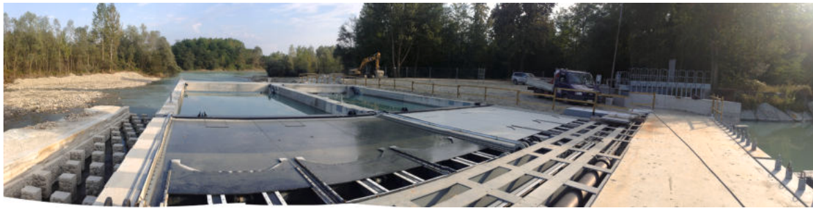
Fig. 15. VLHT installation in the canal, Mazzè, Italy.
